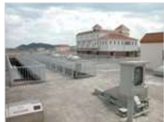
Electrical instrumentation systems for water and sewerage
