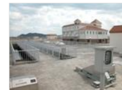
Electrical instrumentation systems for water and sewerage
