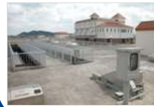
Electrical instrumentation systems for water and sewerage
