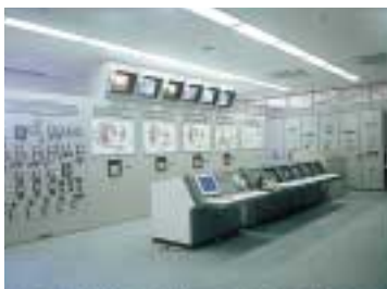
Central monitoring system for incinerating plant
