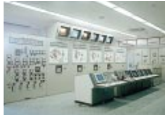
Central monitoring system for incinerating plant
