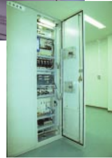
Central monitoring system for sewage treatment plant
