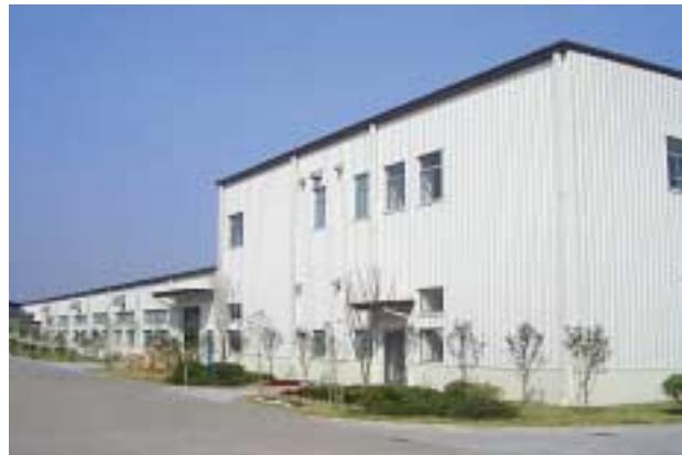
The New Factory
