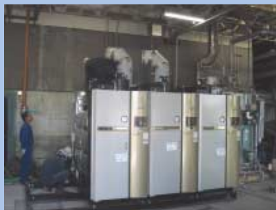
Installation of LPG-fired Boiler
