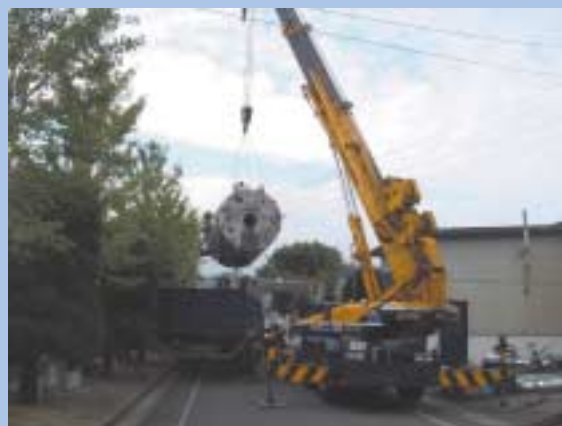
Removal of Oil-fired Boiler
