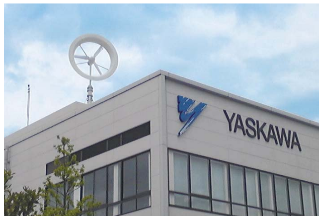
The wind lens turbine power generation system on the roof of the Drive Center
