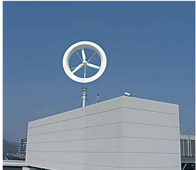
The wind lens turbine power generation system on the roof of the Drive Center
