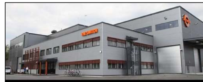
The Switch Engineering Oy
