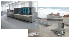
Electric instrumentation systems for water and sewerage
