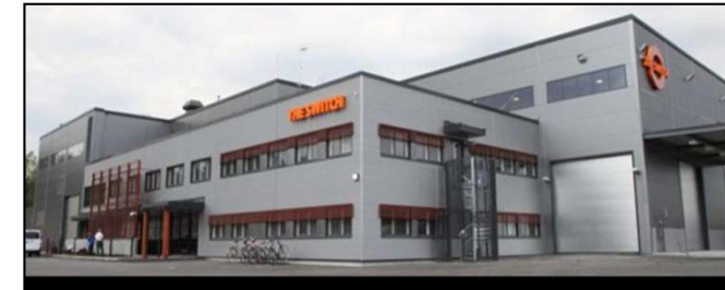
The Switch Engineering Oy
