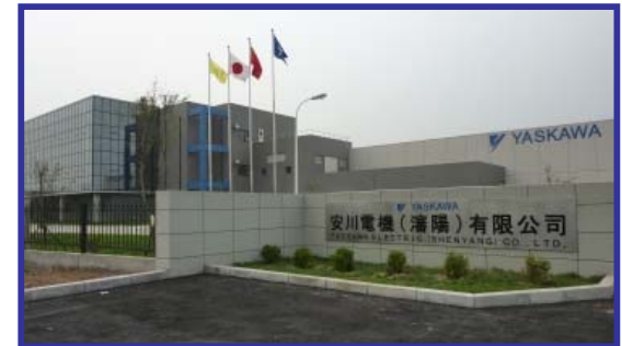
YASKAWA Electric (Shenyang) Co., Ltd
