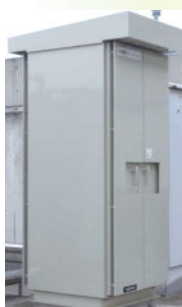
Wind power conditioner*2 installed on a rooftop
