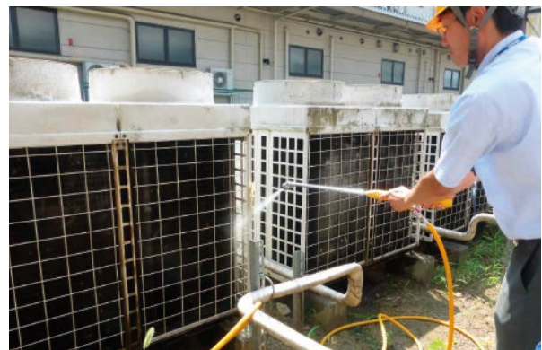
Air conditioning heat exchangers are cleaned
