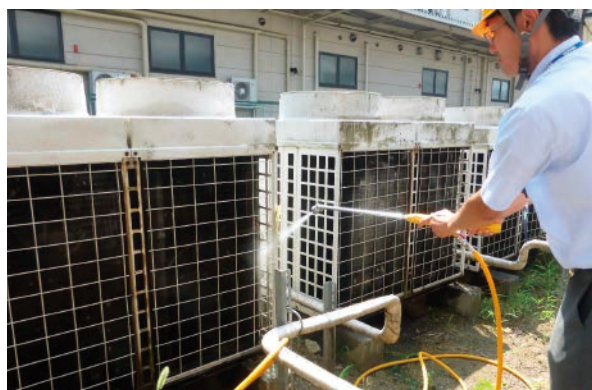
Air conditioning heat exchangers are cleaned
