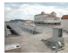
Electrical instrumentation systems for water and sewerage
