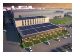
Welfare facility at Yukuhashi plant with photovoltaic generation facility
