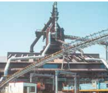
Blast furnace facility
