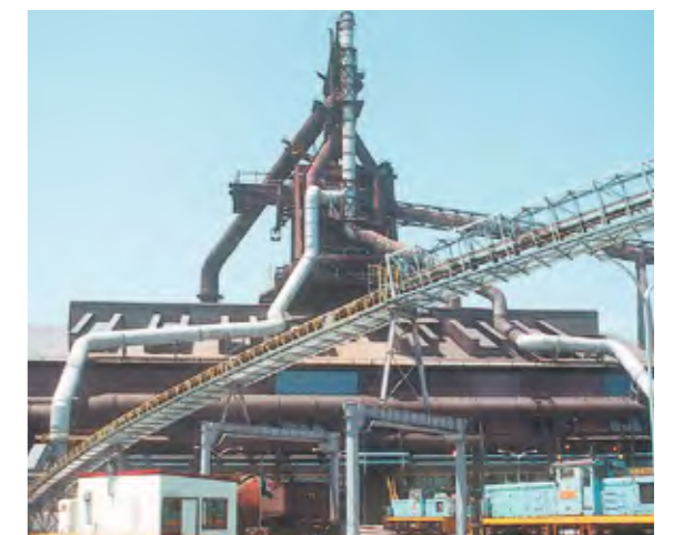
Blast furnace facility
