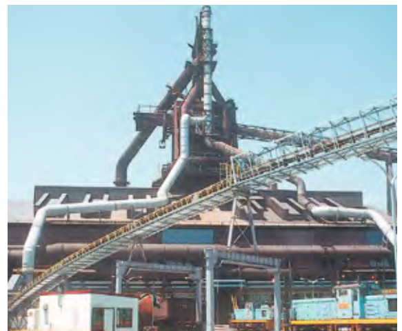
Blast furnace facility
