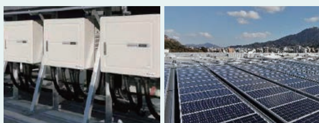
The Enewell-SOL P2 (left), PV inverter manufactured by Yaskawa and 295kW solar power generation system (right) installed on YASKAWA Technology Center which opened in FY2021
