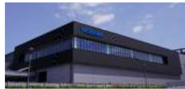
Exterior view of Robot Plant No.5
