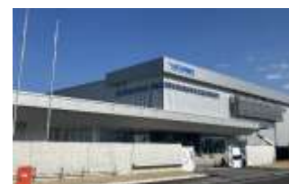
Newly established Minamiyukuhashi Plant
