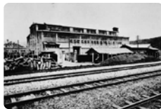
Factory exterior (1919 – Kitakyushu City)
