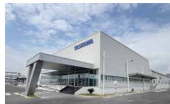
Vietnam PCB Plant
